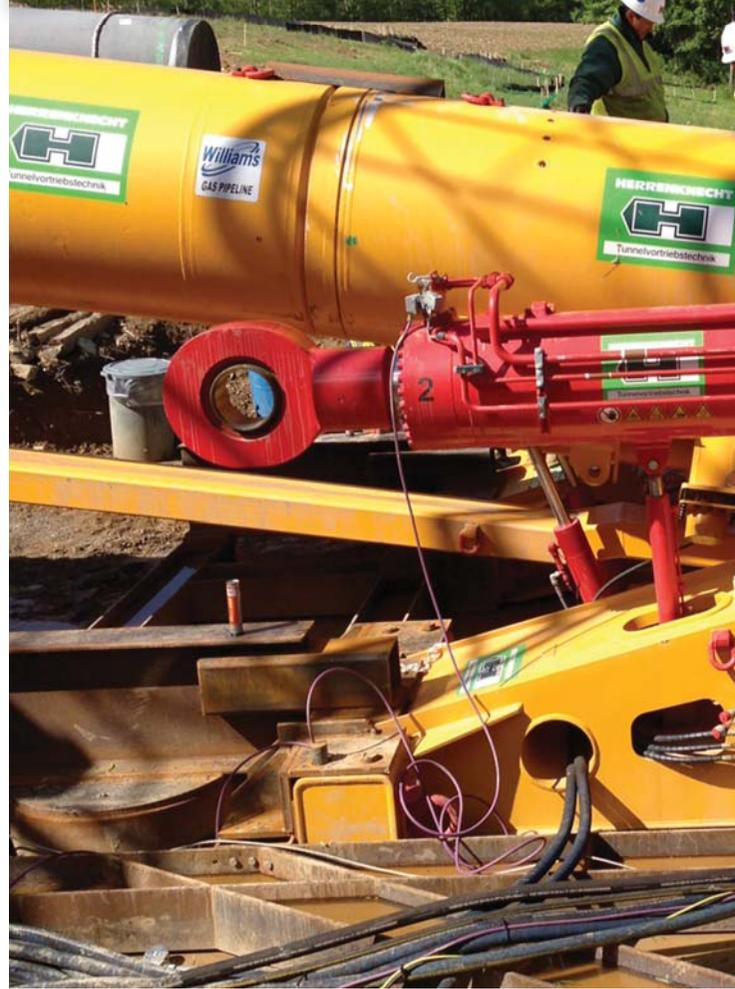
explained. “Then the pipe thruster and launch cradle were placed on the foundation. The DP machine components were assembled on the launch cradle. After the DP machine was completely assembled, the umbilical hoses and pipes were assembled inside the product pipe and welded to a transition piece attached to the TBM.”
